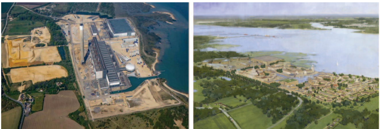
Figure 6: Fawley Waterside – from a 1960s power station to an intelligent merchant city (courtesy Fawley Waterside)
