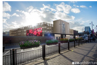
Holmeside Car Park
